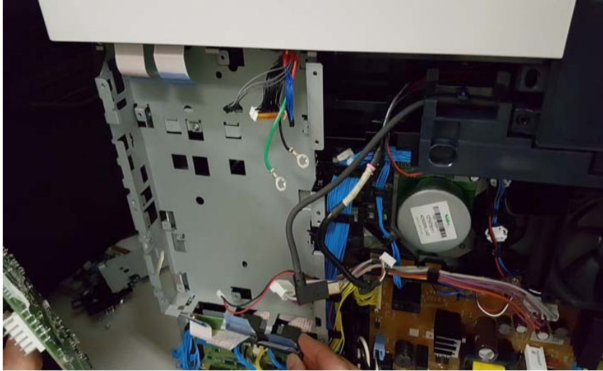
Figure 8 Removal Complete with FCC Guides Remaining In-place
