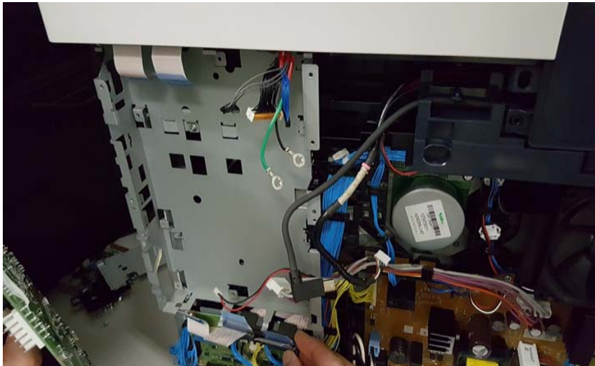
Figure 7 Removal Complete with FCC Guides Remaining In-place
