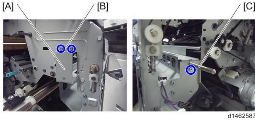
10. Insert and attach the guide plate [A] from the rear (⚙️x2).
