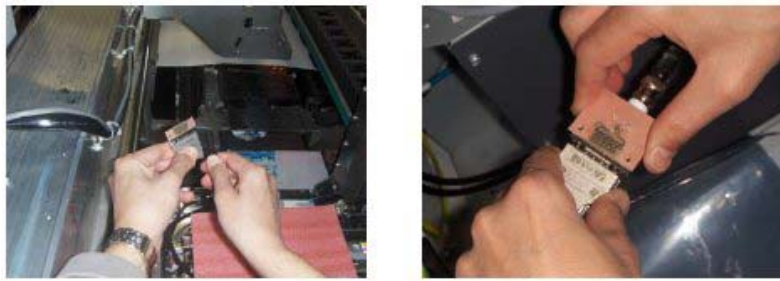
Stressing the 'I' Cable
